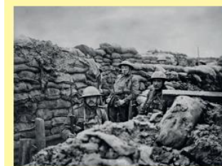
Sandbags form the trench wall
